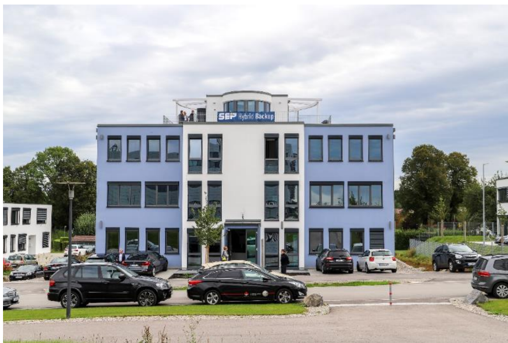
The SNAP Partner Days 2017 were hosted at the newly built headquarters of SEP AG in Holzkirchen
